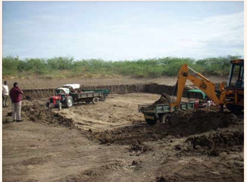
Above: Excavation for a new ooranie. Bottom right: A group of elders
